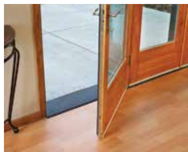
ADA-compliant sill for entrance doors
