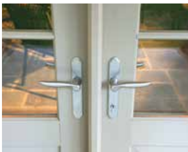
Lever handles in a variety of styles for swinging doors
